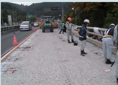
(床版切削状況)
