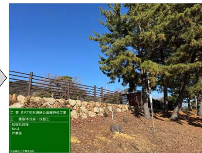
枯損木の伐採①
