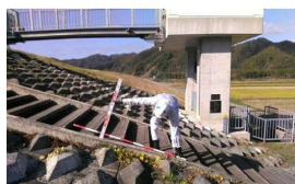
堤防、護岸の点検
