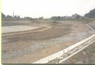
新足羽川堰堤下流
