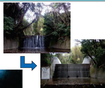
Masonry dam reinforcement
