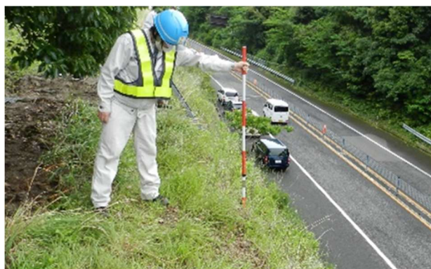
切土のり面の点検
