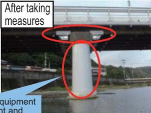
Implementation of equipment for pier reinforcement and preventing falling bridge
