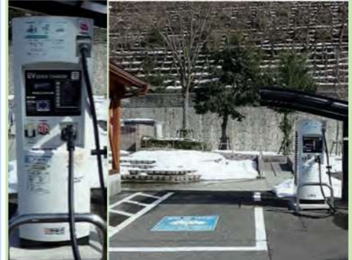
Status of EV charger installation at Roadside Station Kono
