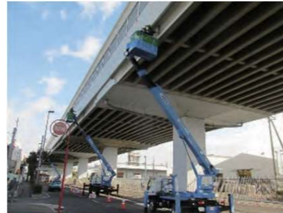
Example of bridge inspection
