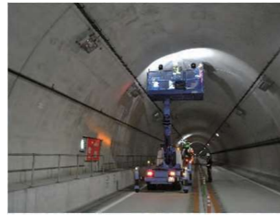
Example of tunnel inspection
