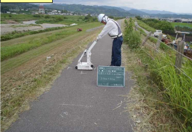
堤防空洞探査
