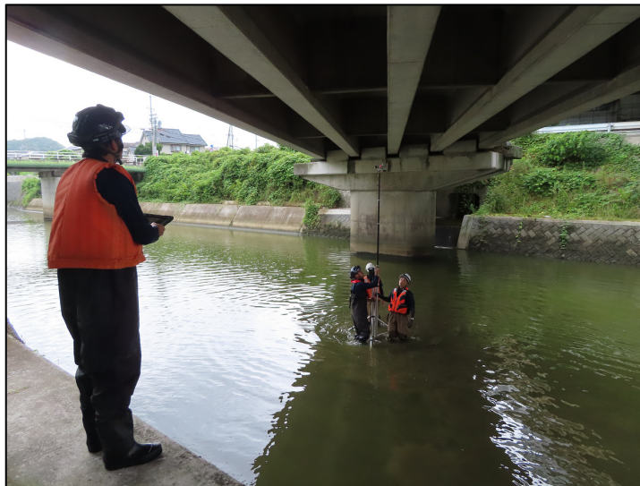
写真-1 点検状況[カメラ設置]
