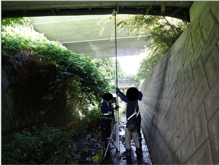
写真-1 点検状況[カメラ設置]
