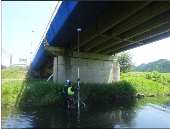
写真-1 点検状況[カメラ設置]
