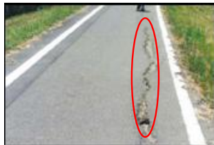
堤防天端の亀裂
