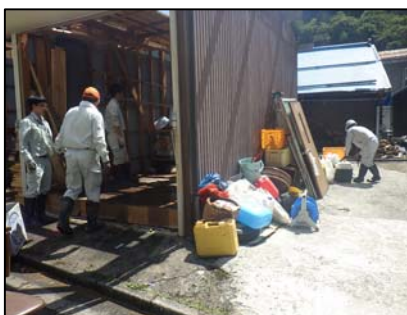
写真-12 H30.9被災家屋の復旧
