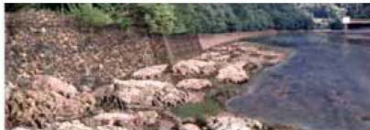
掘削時の状況[平常時流量(約40m 3 /S)]
