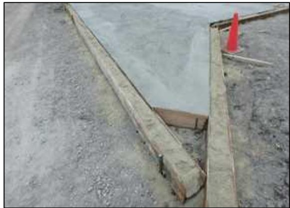
写真-3.2.2 H形鋼型枠
