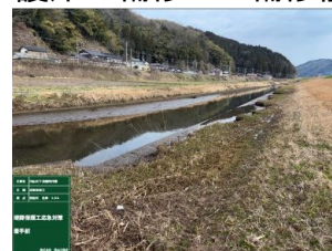
護岸の補修 補修前
