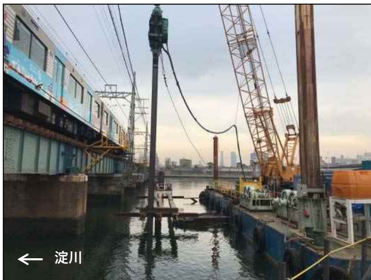
①仮栈橋構築工
