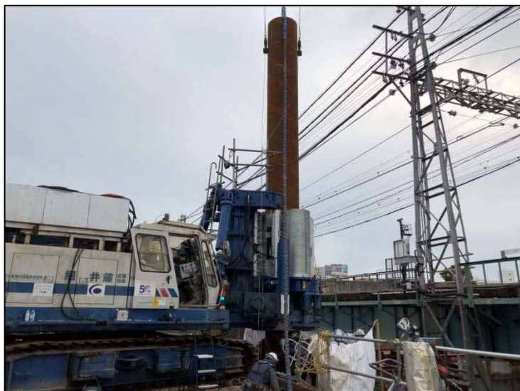
②既設橋梁補強工
