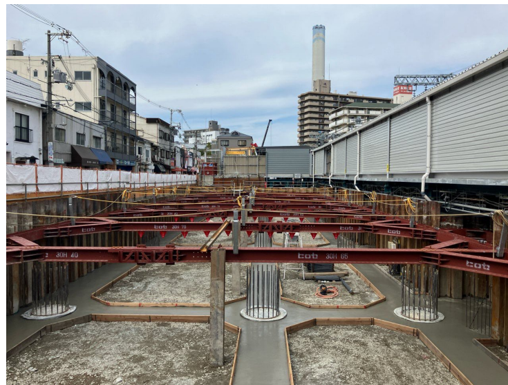
②躯体構築工
