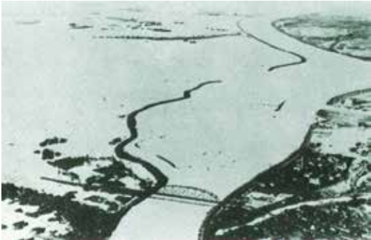
Levee breach at Mukaijima on the Uji River caused by Typhoon No. 13 in 1953
