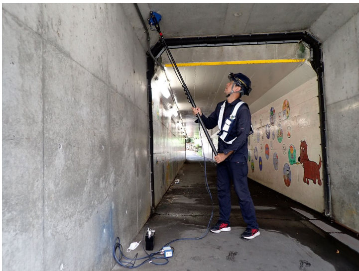
写真-1 点検状況[ハンチ部]
